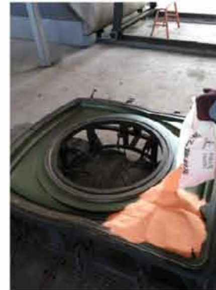
1. Pouring into mould
